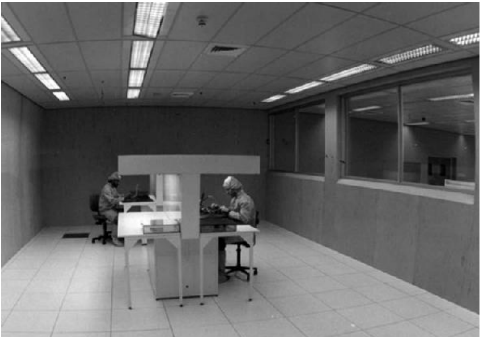
Figure 4. Clean room in the ADVENA Nuclear Weapons Facility. Source: Institute for Science and International Security
