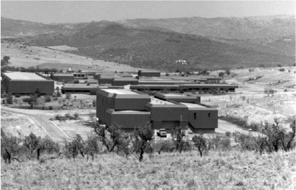
Figure 3. The ADVENA Nuclear Weapons Facility completed just before the termination of the Program. Source: Institute for Science and International Security
